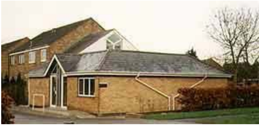
The new Doctors Surgery – at the Western Drive junction with Castlethorpe Rd
