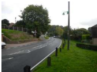
Marquis Car Park Entrance on blind bend
