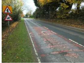
Grass verge with no footpath, backed up on far side. Worn road surface at bridleway crossing point.
