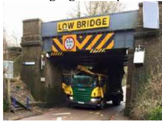
Bridge Collision Kearsney.
