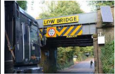
Bridge Collision Kearsney.
