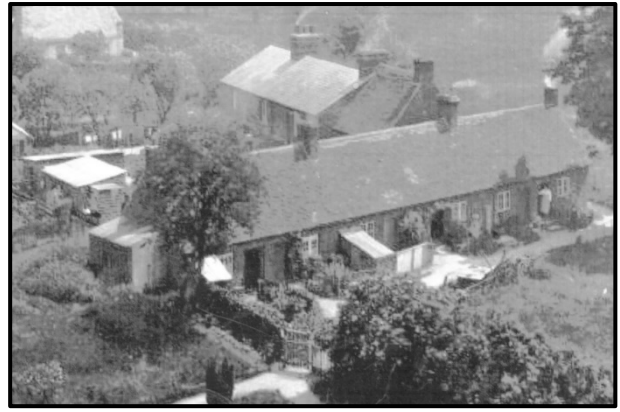
The former Alms Houses at the top of Church Lane with at least one house. Whaddon CofE school shown very top left.
