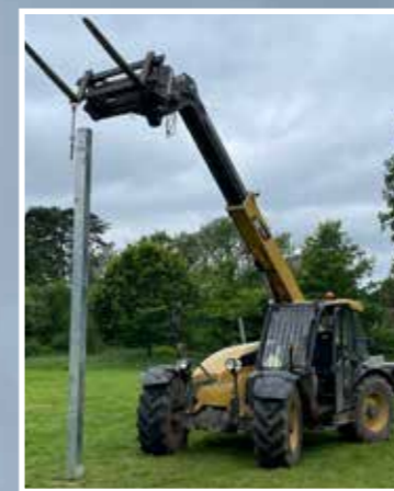
Going up: Matthew Price drops the post into the ground
