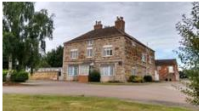
Broughton Grange, Broughton (building) is operated as office premises
